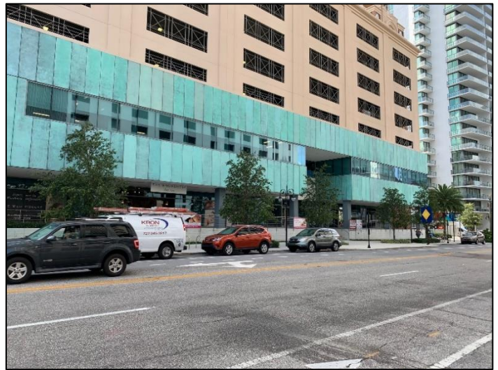
Building Entrance (Looking North)
