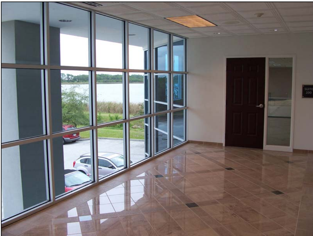
SECOND FLOOR LOBBY
